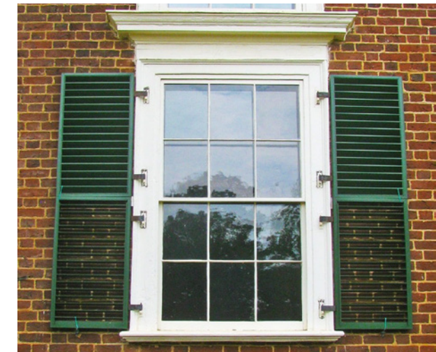
Green louvered shutters add interest by contrasting the red brick.
