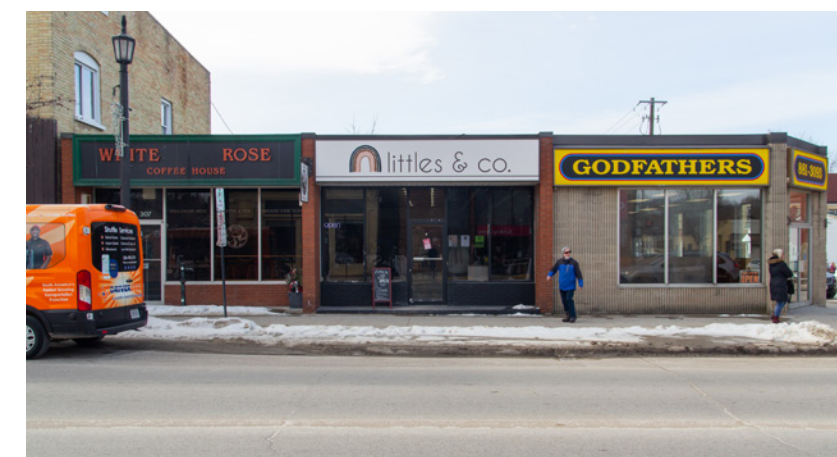
Existing Façade, March 2023
