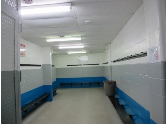
North Dressing Rooms – Still with T12s should be converted to T5's.
