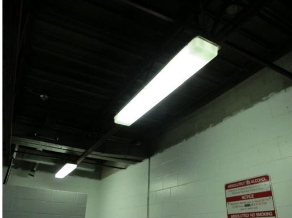
North Dressing Rooms – Still with T12s should be converted to T5's.
