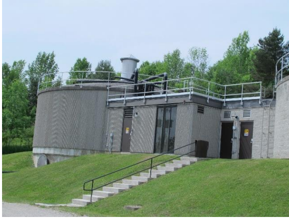
The Digester is the final stage of anaerobic digestion that produces methane for use in the gas generator.
