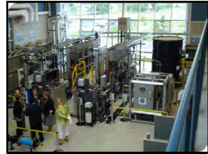
The Walkerton Clean Water Centre (Source: Infrastructure Ontario).
