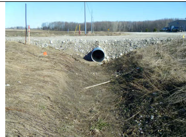
PLATE 4 NEW DRAINAGE UNDER NEW GRAVEL ENTRANCE
