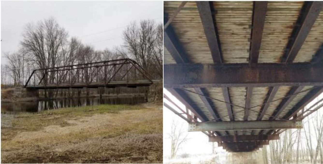
Riversdale Bridge – BCI: 33
