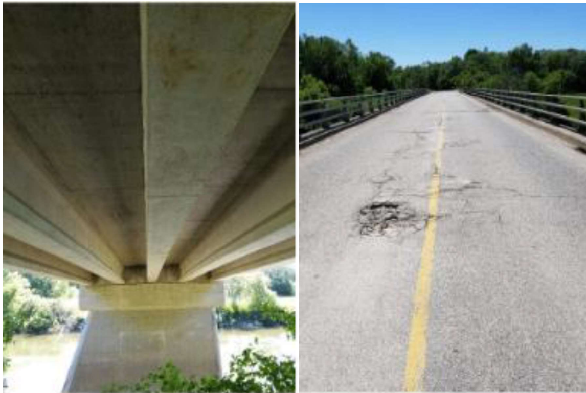
Weis Memorial Bridge – BCI: 65
