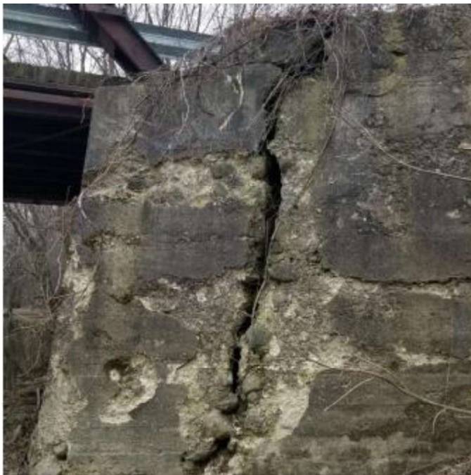
Riversdale Bridge – BCI: 33
