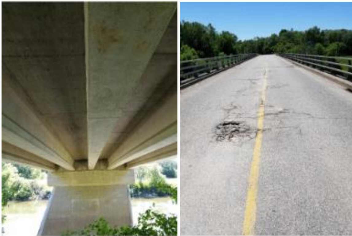
Weis Memorial Bridge – BCI: 65
