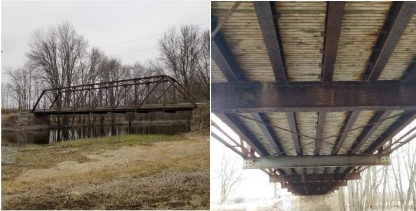
Riversdale Bridge – BCI: 33
