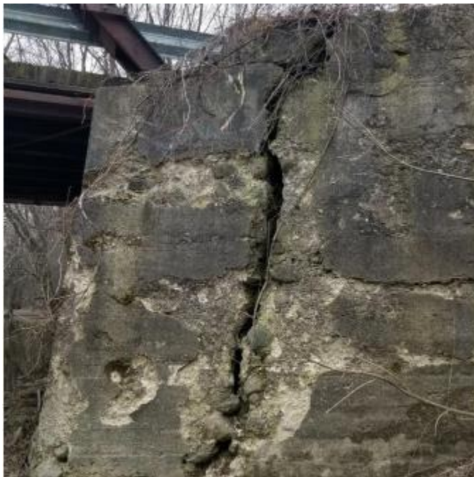
Riversdale Bridge – BCI: 33
